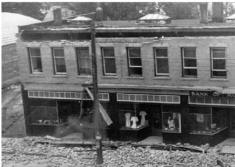
The 1946 earthquake on Vancouver Island substantially damaged homes, businesses and roads.
